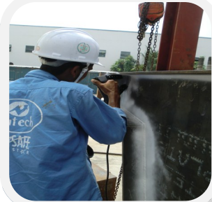
Magnetic Particle Testing
